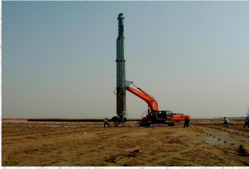
Fig. 2 Typical PVD Installation stitcher
